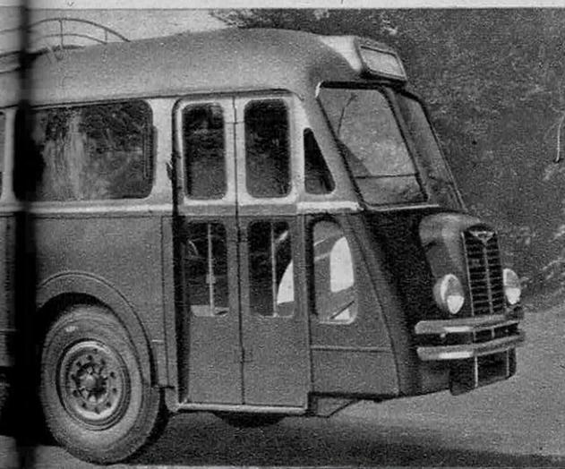
DIESEL 85 CH A L'AVANT. CAISSE MONOCOQUE
