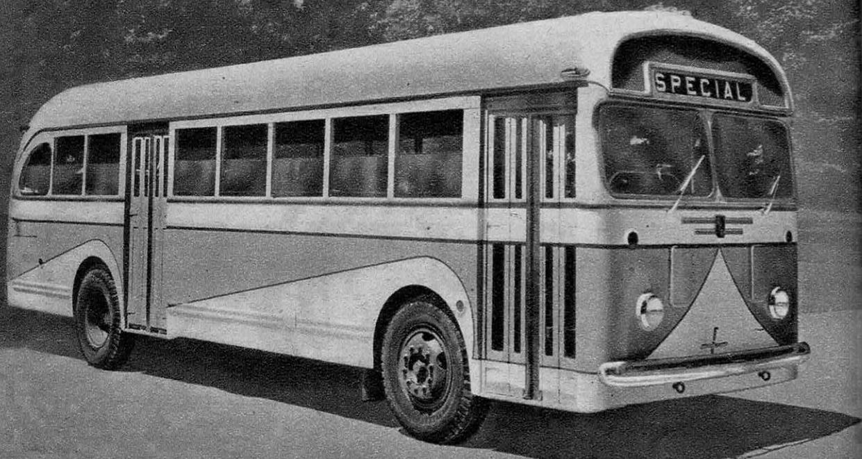
AUTOBUS REO, 33 PL. MOTEUR A ESS. 127 CH. MONTÉ HORIZONTELEMENT AU MILIEU DU CHASSIS.
