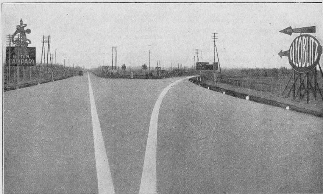
UNE BIFURCATION SUR LA ROUTE SPÉCIALE POUR AUTOMOBILES DE MILAN AUX LACS EST EN BÉTON DE CIMENT AVEC ENDUIT DE BITUME
