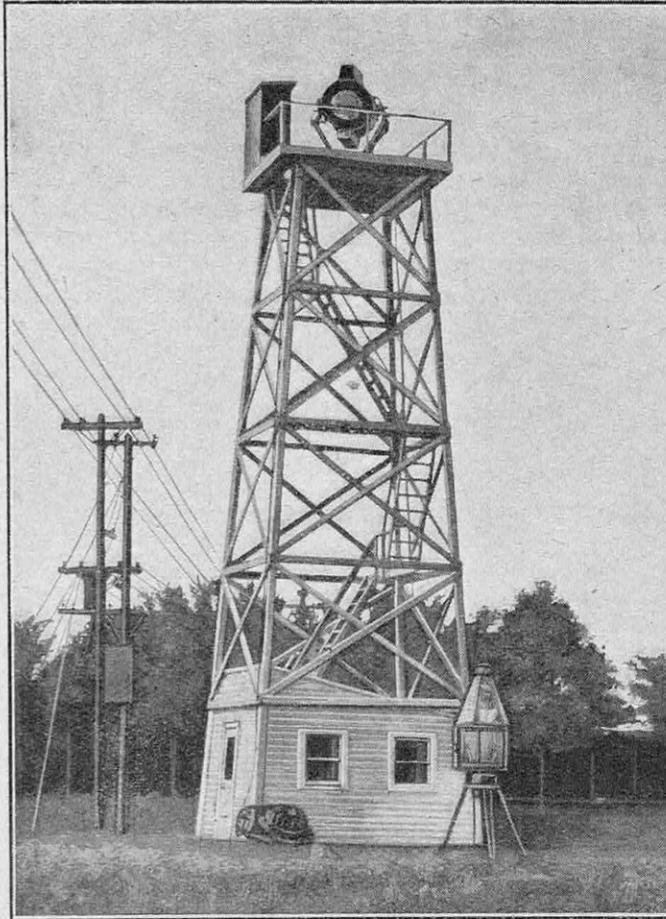
CE PROJECTEUR, MONTÉ SUR PYLONE, EST VISIBLE DANS UN RAYON DE 250 KILOMÈTRES
