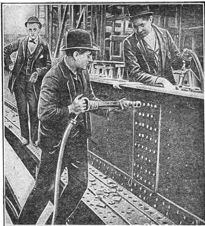
POSE DE RIVETS AU MOYEN D'UN MARTEAU PNEUMATIQUE
