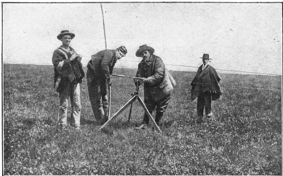
MESURE D'UNE BASE GÉODÉSIQUE AU MOYEN DU FIL JADERIN
