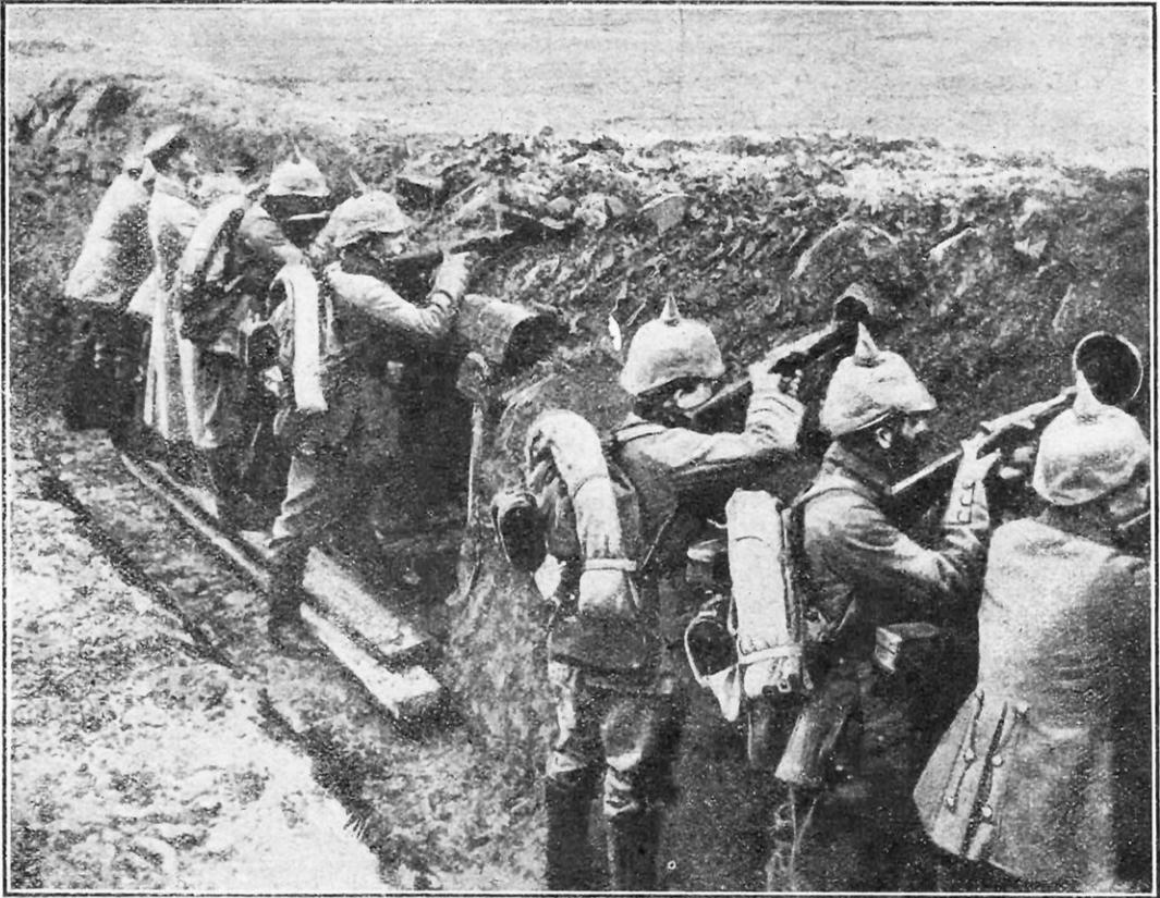
FRANCHÉE AVEC PARAPET EXHAUSSÉ MUNI DE CRÊNEAUX EN POTERIE
